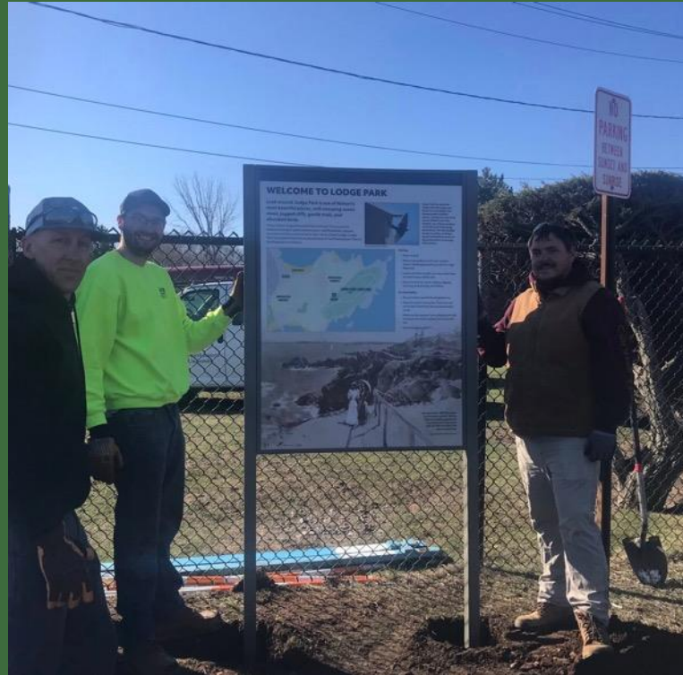
DPW crew installs interpretive panel
